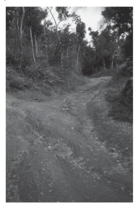
Figure 2. A typical steep road segment near Bordeaux Mountain with a deeply rilled travelway.
